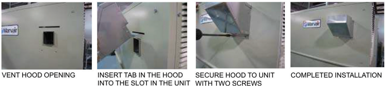
Figure 6. Vent Hood Installation
