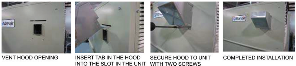
Figure 6. Vent Hood Installation
